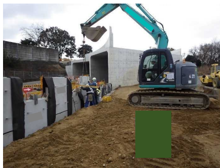
壁面材組立て
