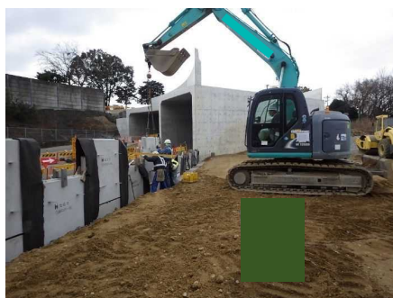
壁面材組立て
