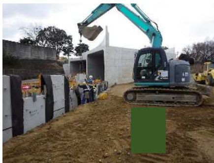
壁面材組立て
