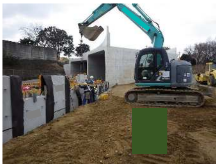
壁面材組立て
